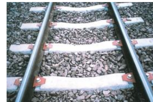
Railtech Rail Fastening Clip
